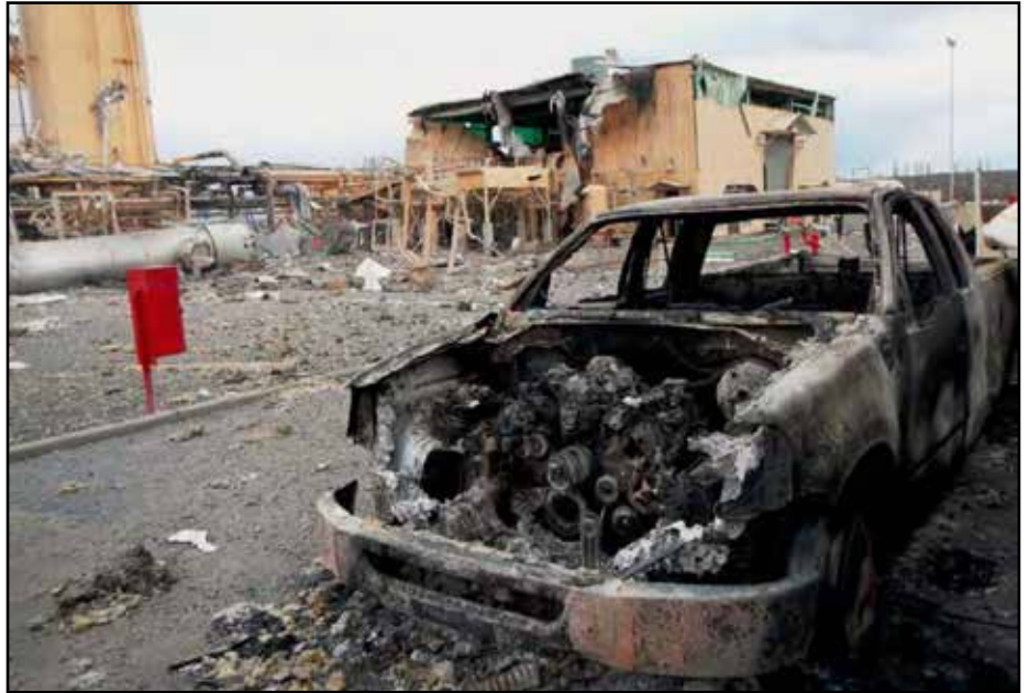
An explosion at a liquefied natural gas (LNG) plant in eastern Washington forced hundreds to evacuate their homes, injured five workers, and caused $69 million in damages. It was one in a string of accidents at The Williams Companies' natural gas facilities that in the last five years has killed five workers and injured at least 120 people. Photo: via Sightline Institute
