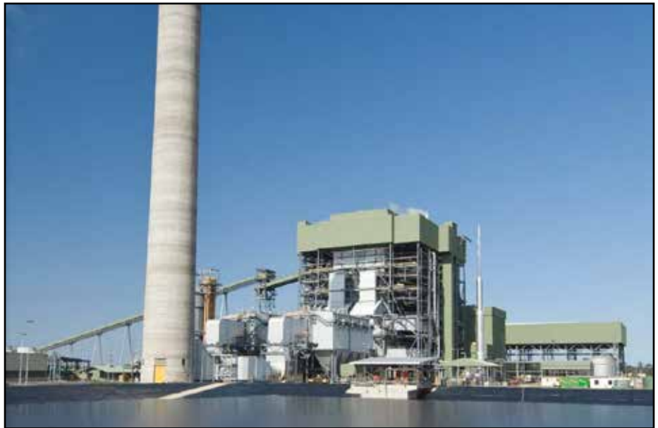
Australian's newest coal fired power station at Kogan Creek, Qld, opened in 2007. Coalition politicians are pushing to build more coal fired plants despite cheaper renewables and the danger for climate change. Photo: CS Energy
