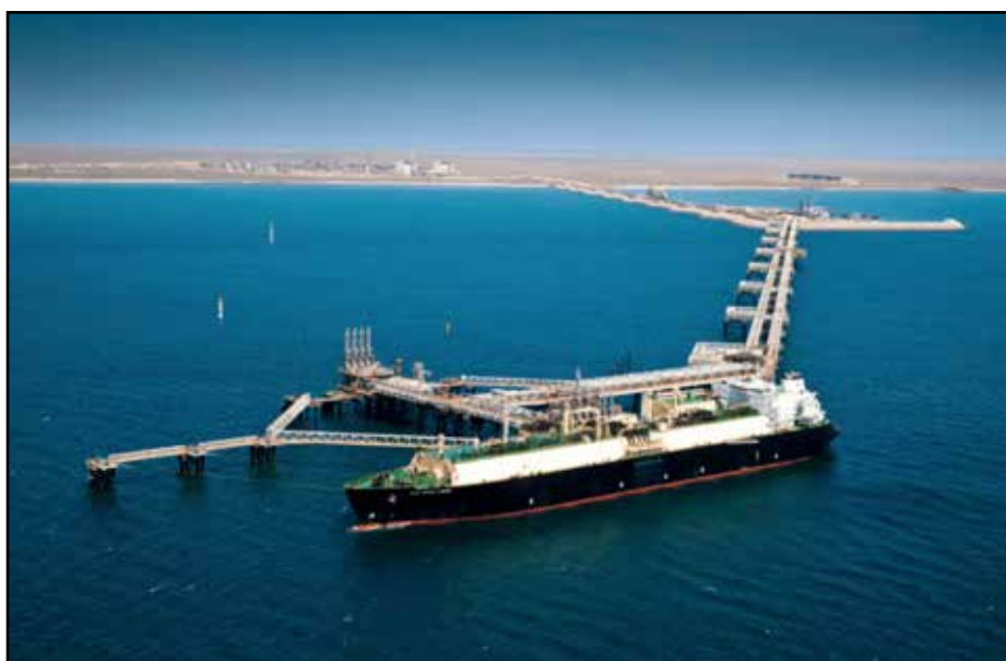
Chevron's Gorgon LNG project on Barrow Island, WA. The company's carbon capture and storage program, a critical factor in the project's approval, is two years behind schedule with no sign of getting started. Photo: Chevron
